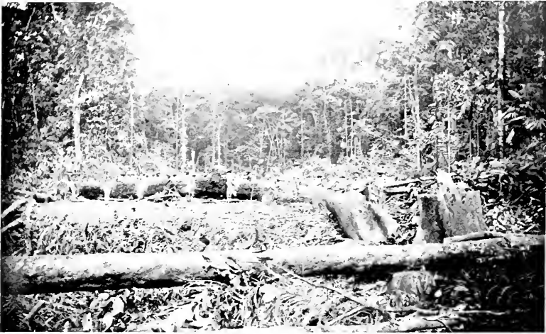
CLEARING THE LINE OF THE RAILROAD.
